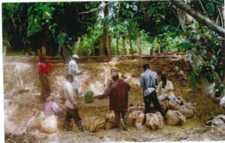
Photo. 3-23. Excavation of river bottom and jute bags
