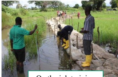
On the job training
