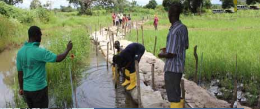
On the job training
